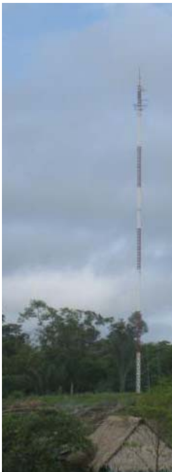
Figure 65. Braced tower.
