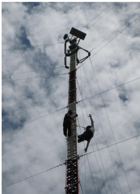
Figure 36. 60 meter tower on San Juan, on the top are installed the telecommunication and energy equipments.
