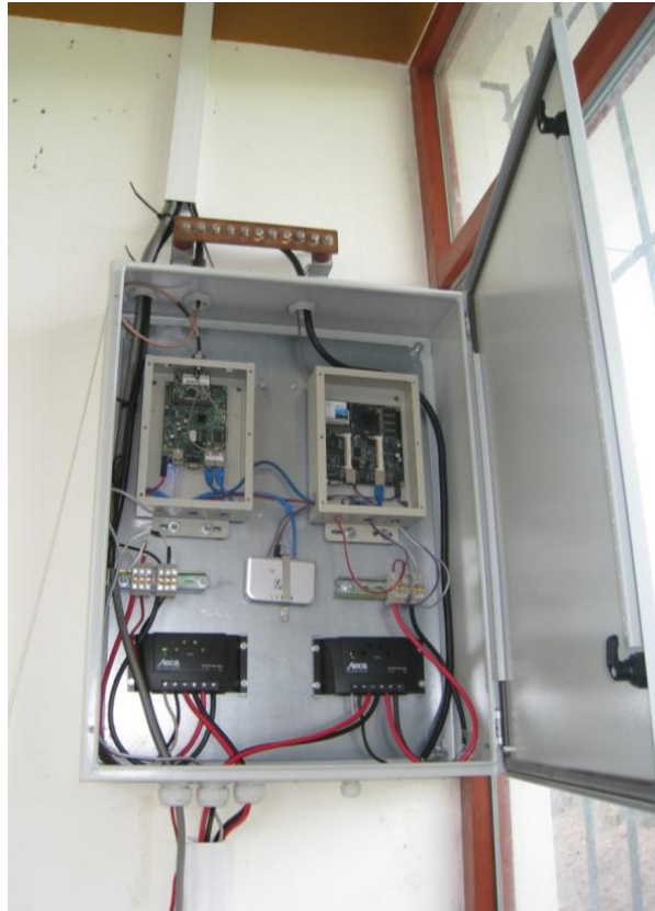
Figure 35. Equipment cabinet in Varadero health post. We can see the router Mikrotik on the left and the VoIP server on the right, below the are two photovoltaic controllers.
