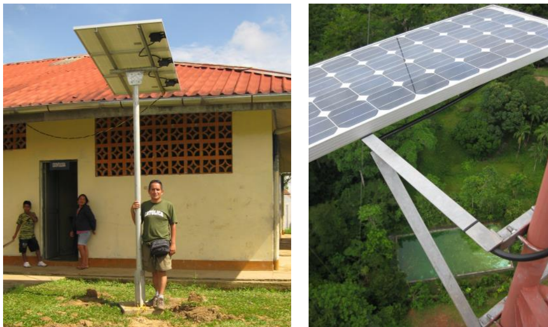
Figure 22. Mechanical support for solar panels.
