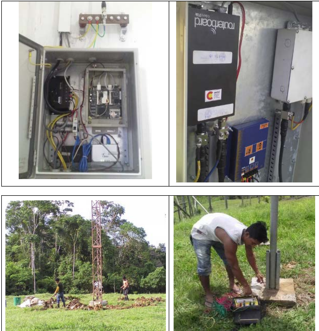
Figure 41: Client station (upper-left corner); repeater station (upper-right corner); Grounding system maintenance at the repeater station (lower-left corner); Grounding system maintenance at the client station (lower-right corner)
