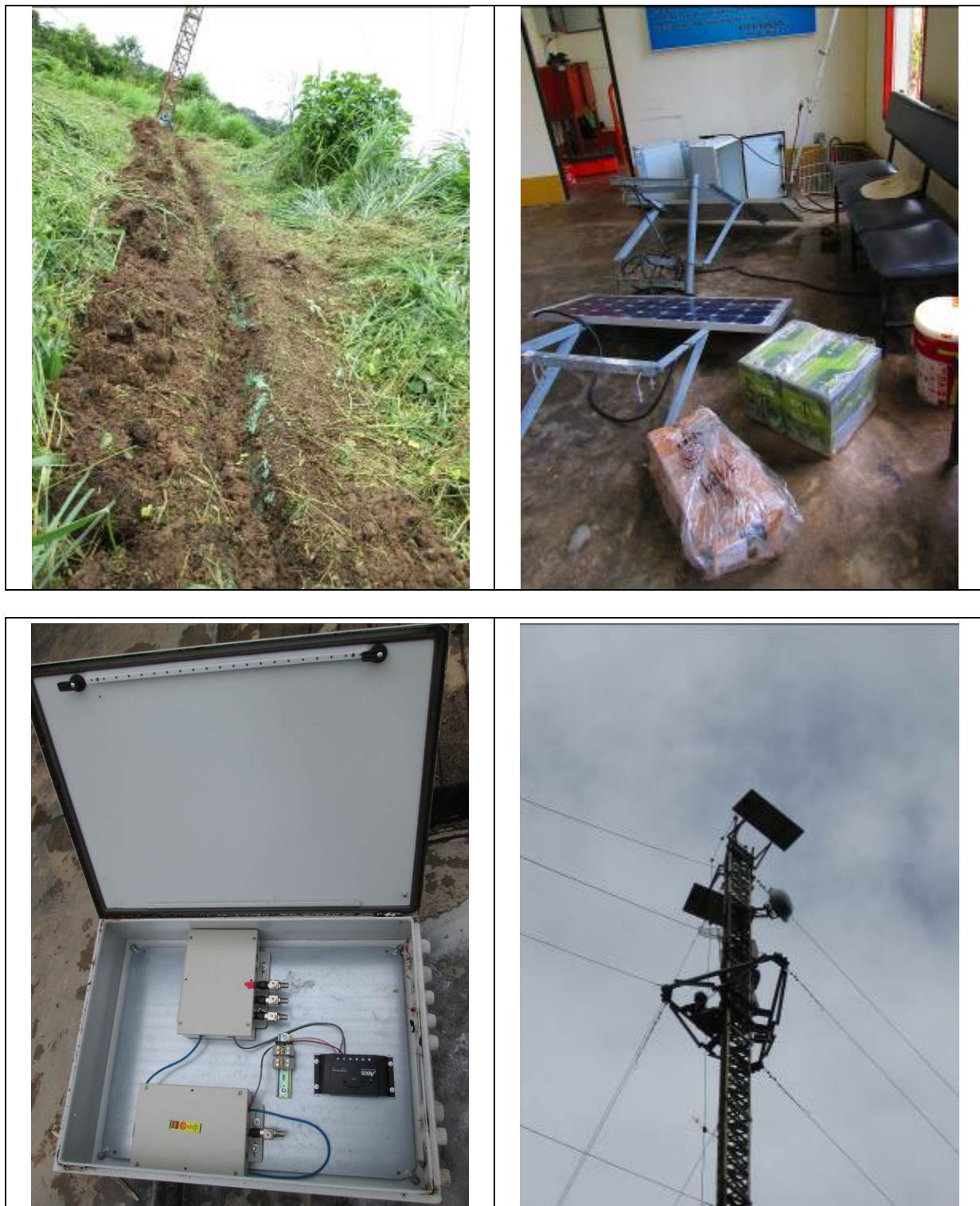
Figure 56: Upgrade of the grounding system and maintenance of the equipment used in the repeater located in San Gabriel de Varadero
