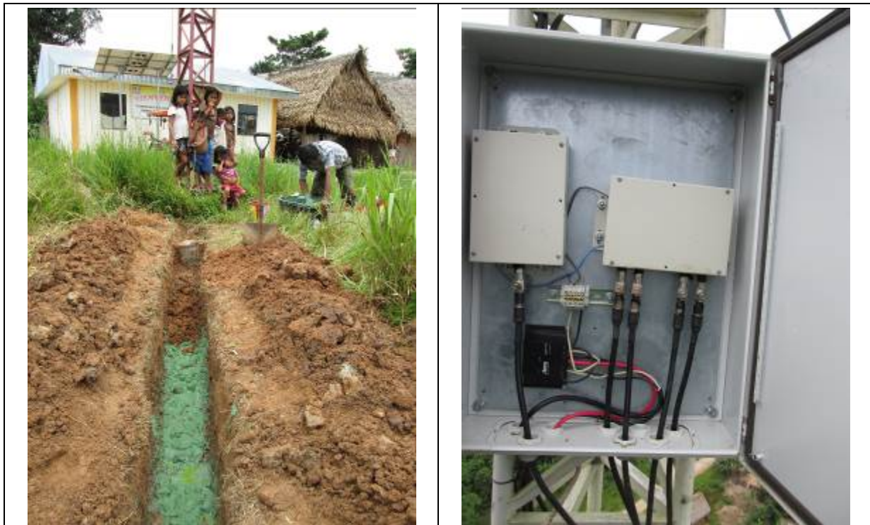
Figure 54: Upgrade of the grounding system and maintenance of the equipment used in the repeater located in Varadero
