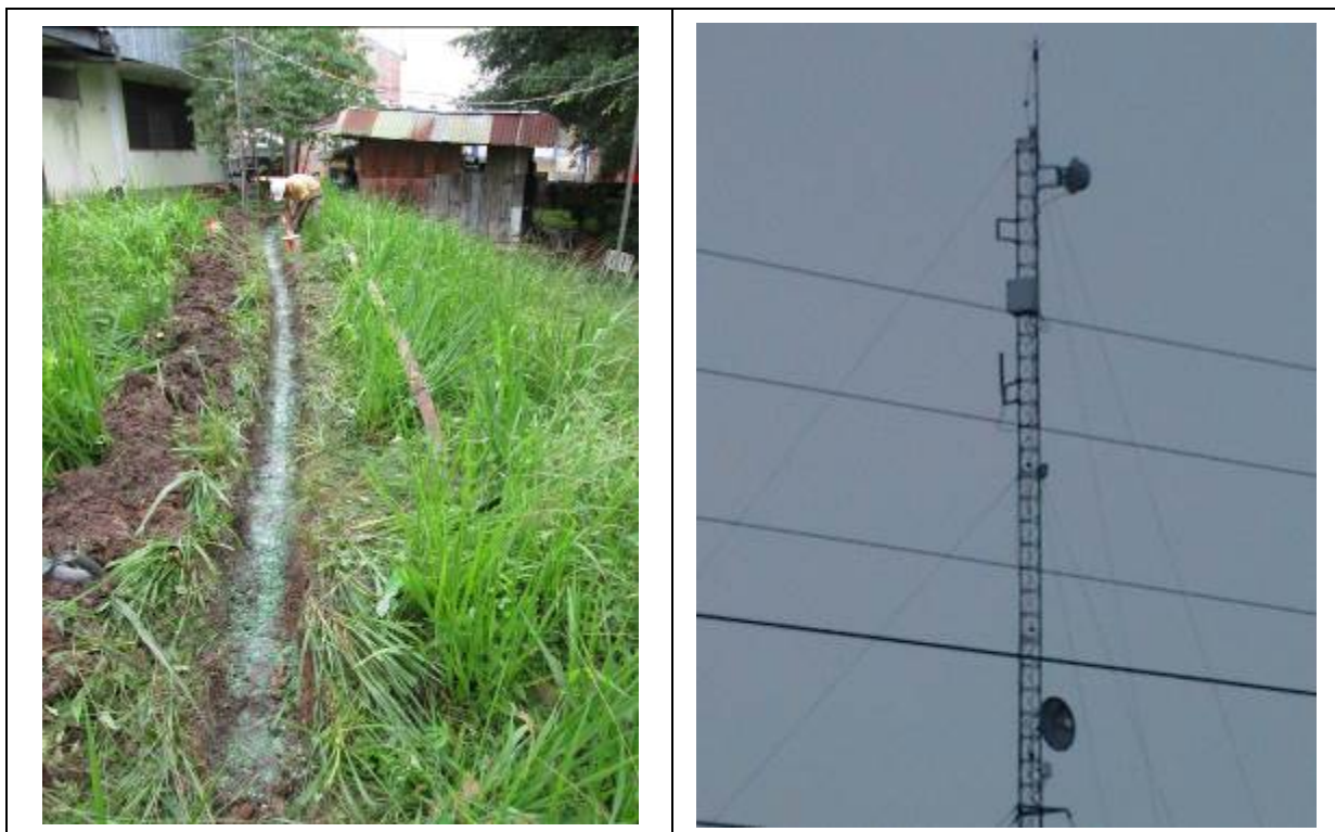
Figure 53: Upgrade of the grounding system and maintenance of the equipment used in the repeater located in Santa Gema Hospital
