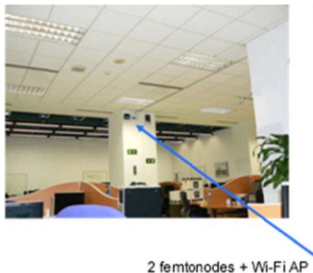
Figure 3.40: Two femtonodes and one WiFi access point installed in one of the office's pillars in TID premises.
