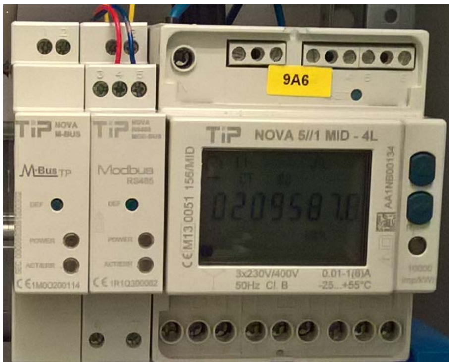
Figure 5: It shows the not connected M-Bus TP device (left), the TIP NOVA RS485 MOD-BUS interface (middle with red and blue power supply cables) and the Mainau AG owned smart meter TIP NOVA 5/1 MID-4L (right).
