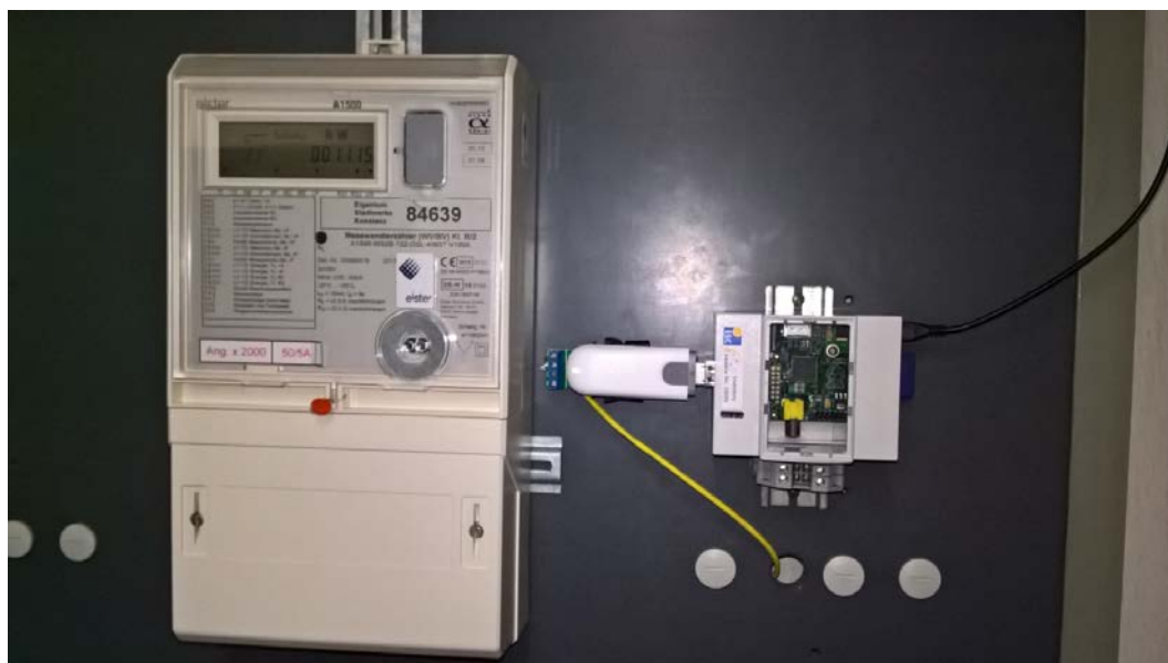
Figure 17: The picture of installation from the 17 th Oct. 2016, when the Raspberry PI-1 is again connected via S0-Interface with the A1500 Elster smart meter in the MV-LV distribution cabinet.
