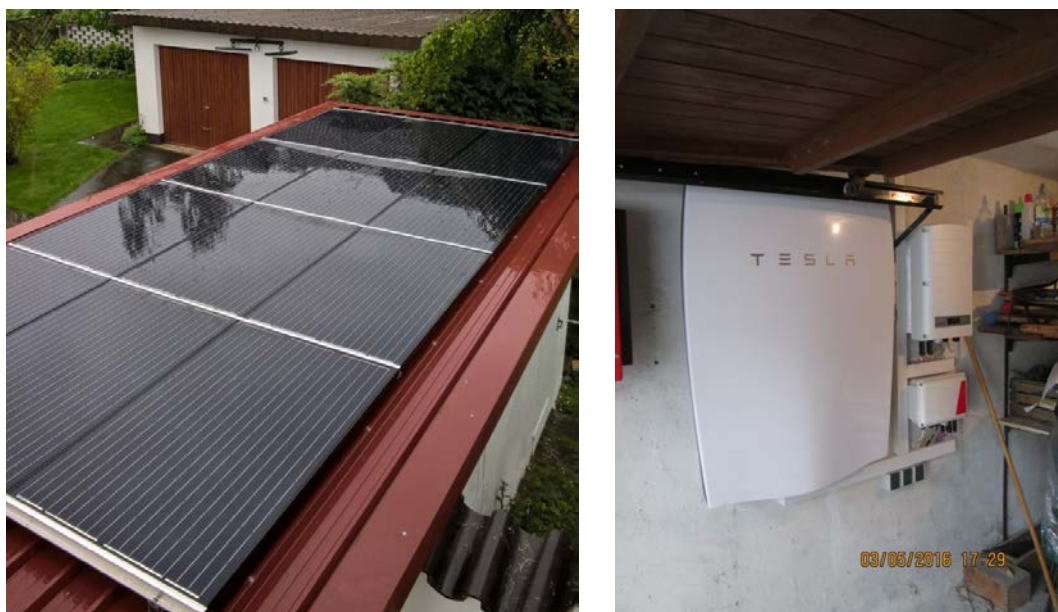
Figure 32: Right: The Tesla Power battery with integrated solaredge™ interface and inverter; left: The flat roof top mounted PV module as recently mounted in May 2016 during the trial period.
