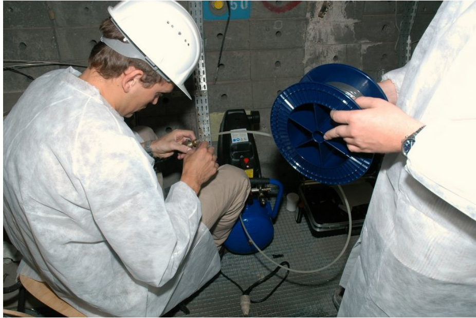
Figure 27: The optic fibres being inserted into the capillary tube using the blow-in method at the CORALUS-4 set-up in the underground laboratory at SCK in Mol
