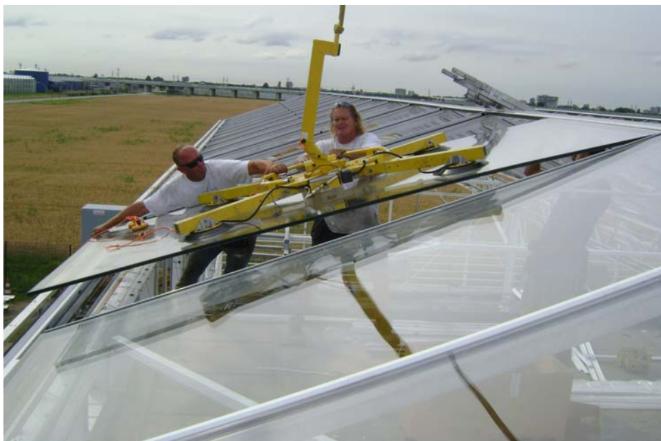
Figure 3. The placing of the innovative double-glass roof on the Venlow greenhouse prototype (co-financed by the Dutch Ministry of Economy and Agriculture and the Dutch Horticultural board). Together with innovative de-humidification, an energy saving of 50% was attained, without loss of production
