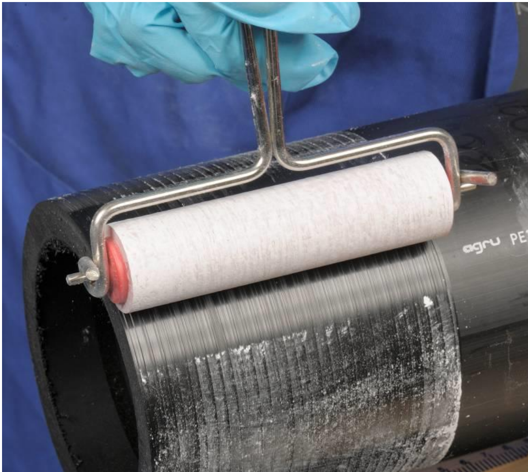
Figure 11 Application of talc on to the pipe surface for EF welding.
