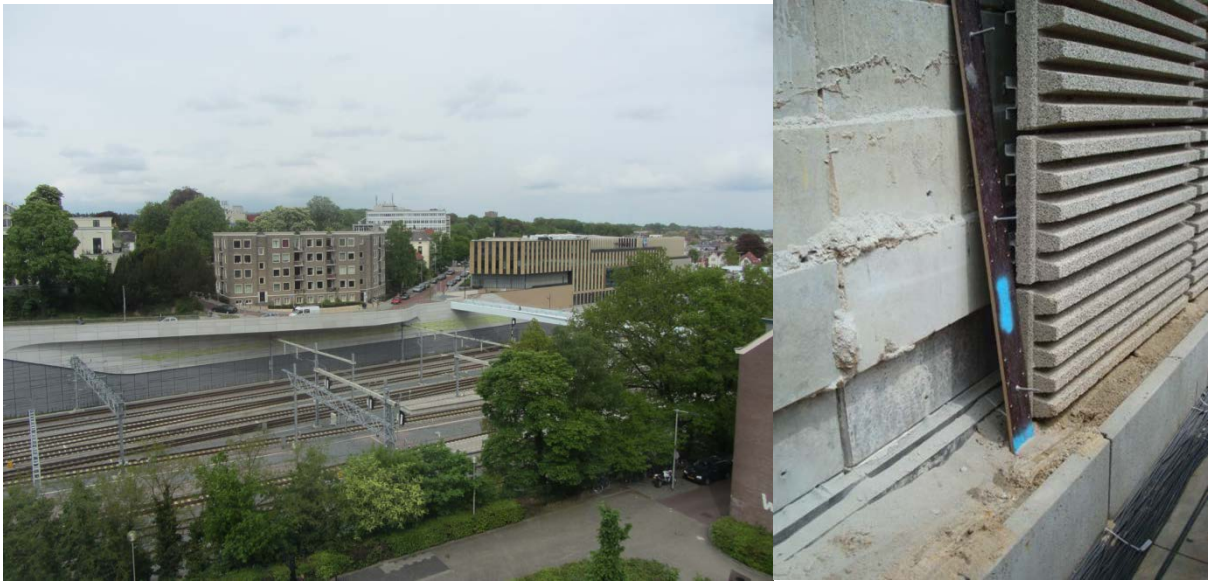
fig. 12: coated ground wall, built in Arnhem, The Netherlands; in the left picture the top of the resilient layer can be seen (two 60 mm black slabs, partially covered with sand), just where the ground wall surfaces and continues as a ground retaining wall (with sound absorbing panels)
