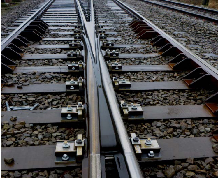
fig. 11: installation of the CDM-Elastiplus system in a crossing in Remersdaal (BE)
