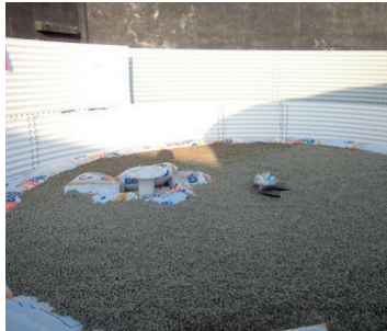
Photo 7. Bulk insulation of the tank bottom
