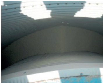
Photo 9. Insulation of the bottom of the STES
