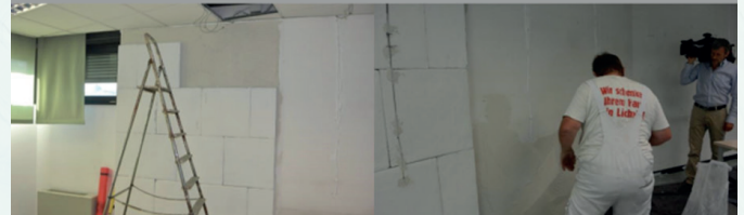
Application of the perlite insulation boards
