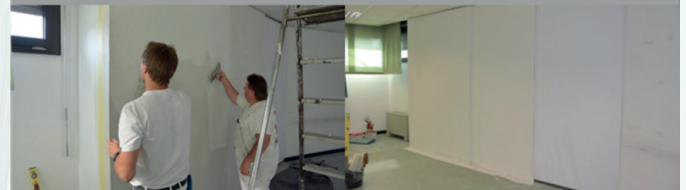
Final finish of the inner retrofitted wall partitions
