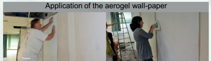
Final finish of the inner retrofitted wall partitions
