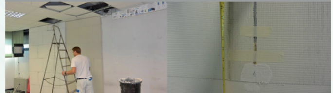
Flat laminated panel with aerogel containing fibrous mat
