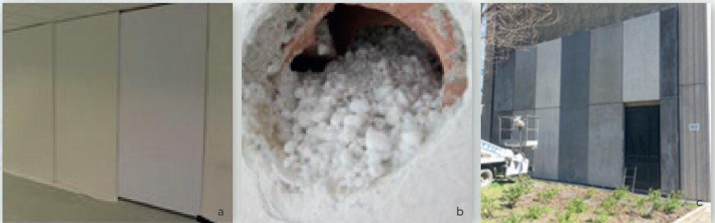
Figure 19: Test facades retrofitted internally (a), in the cavity (b) and externally (c)
