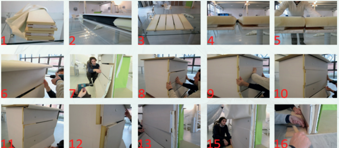
Figure 12: Installation process for aerogel coated solution
