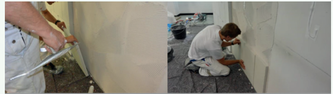
Flat laminated panel with aerogel containing fibrous mat
