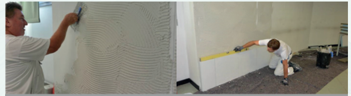
Application of the perlite insulation boards
