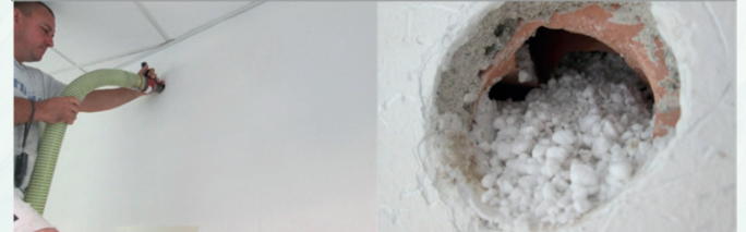
Loose hydrophobic perlite for insulation inside cavity wall
