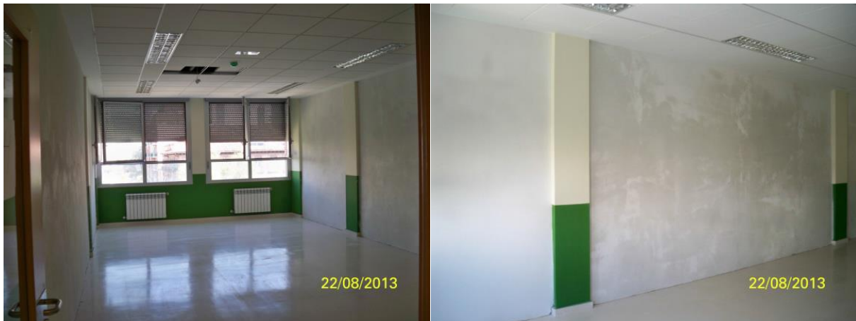
Figure 19: Installed plaster system in the test classroom.
