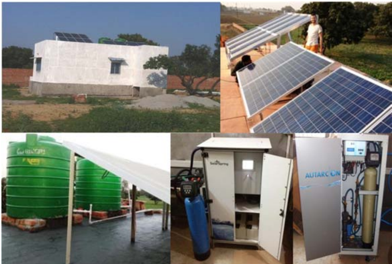
Figure 6: Laboratory building, solar PV panels, water tanks and UV and AO disinfection systems implemented at large AMU pilot plant.
