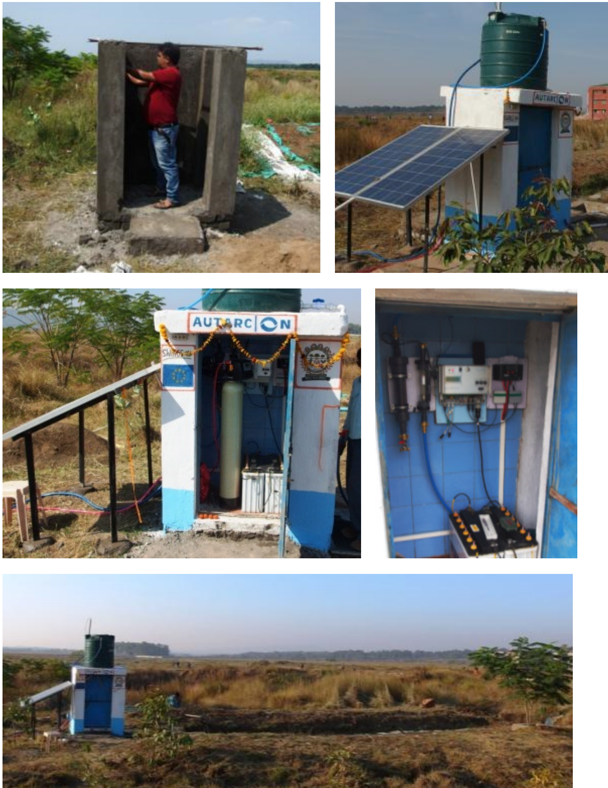
Figure 28: Construction of building for water tank and solar panels and installation of disinfection unit at Amarkantak (IGNTU Campus site).
