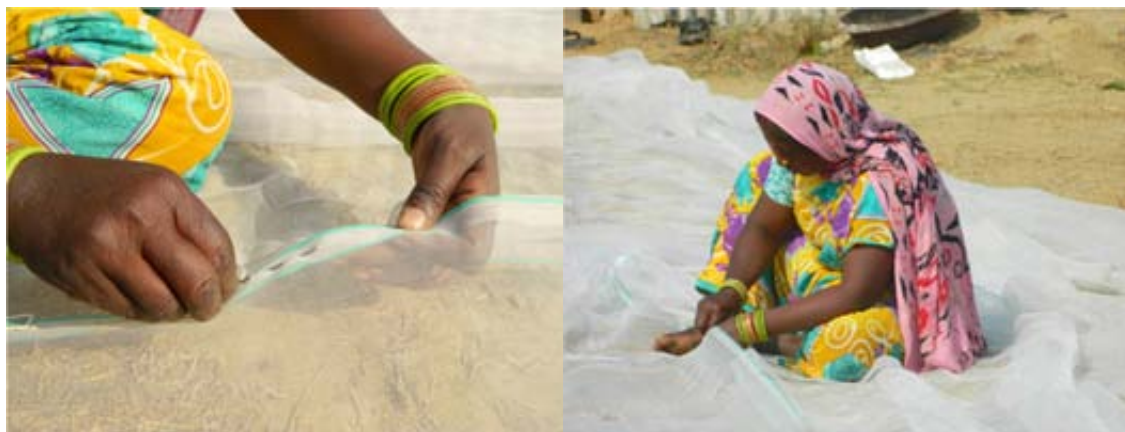
Figure 9: Sewing the geotextile for the VF beds of the FS pilot plant.
