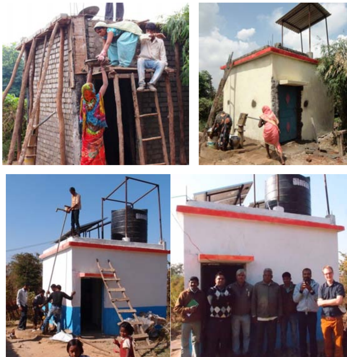
Figure 21: Construction of the water tower structure at Lalpur disinfection pilot plant (IGNTU site).
