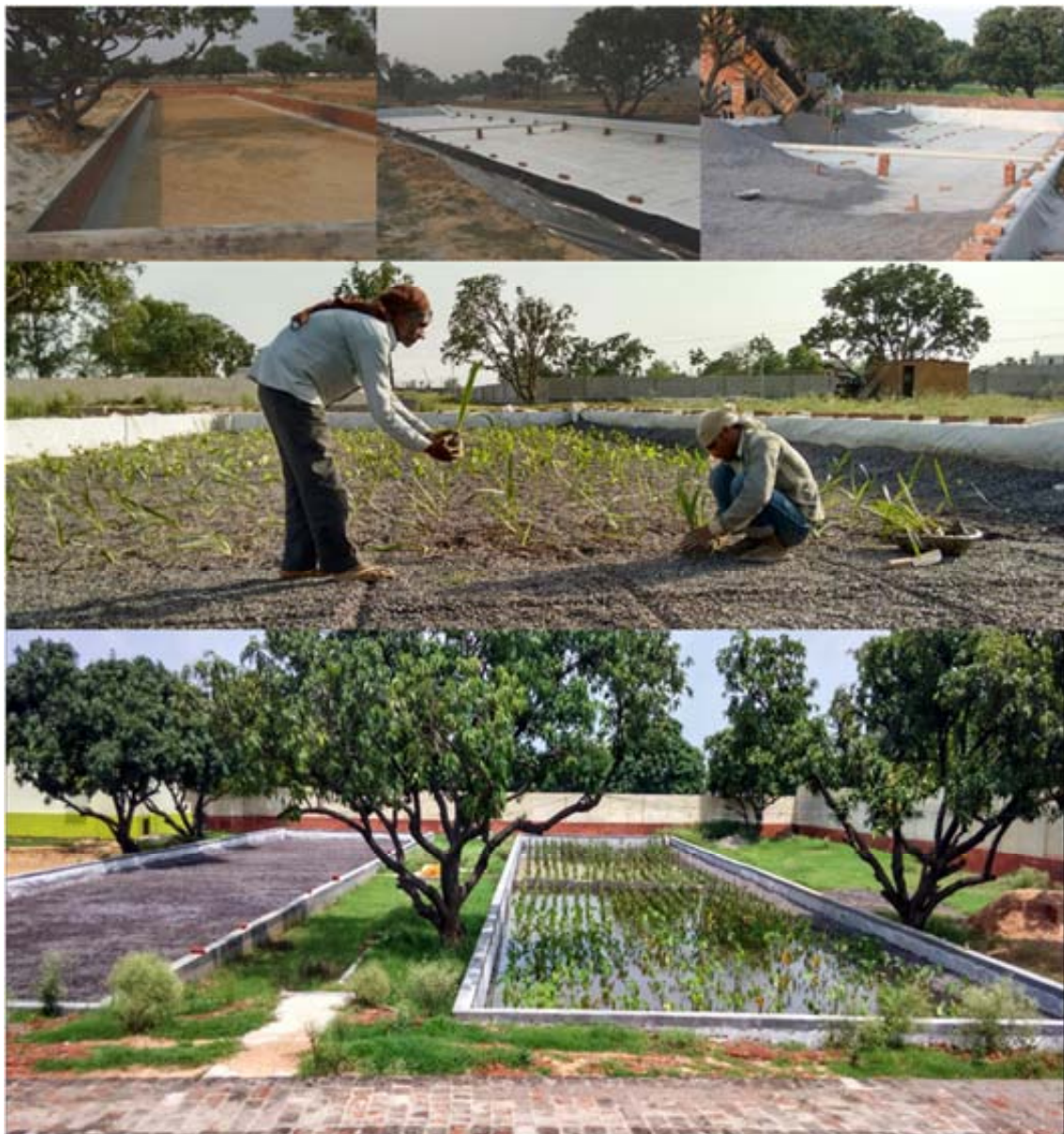
Figure 5: Horizontal constructed wetlands implementation.
