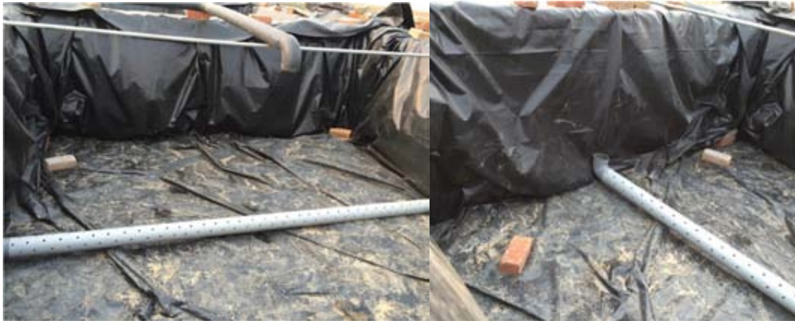
Figure 7: View of the installation of the distribution pipes (left) and the draining pipes (right).
