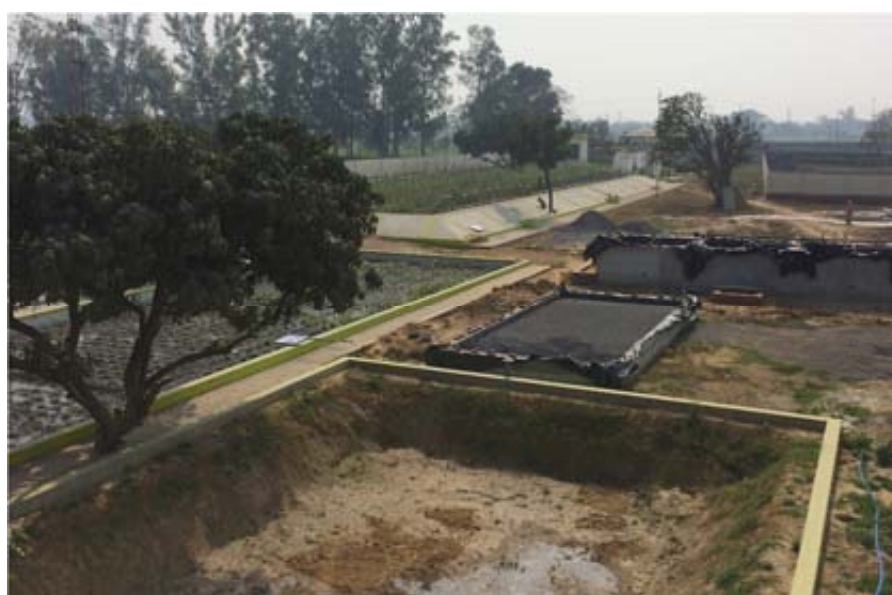
Figure 11: View of the whole FS under construction, including VF bed, HF bed and maturation pond. To the left the large AMU pilot plant in operation can be also observed.
