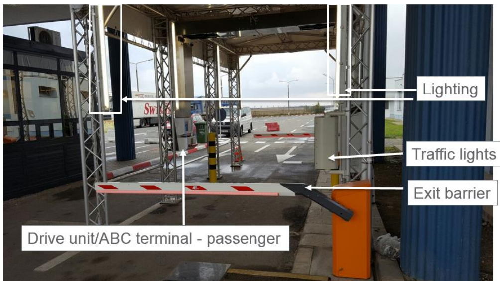
Figure 9: Installation of the land border gate tunnel in Moravita.
