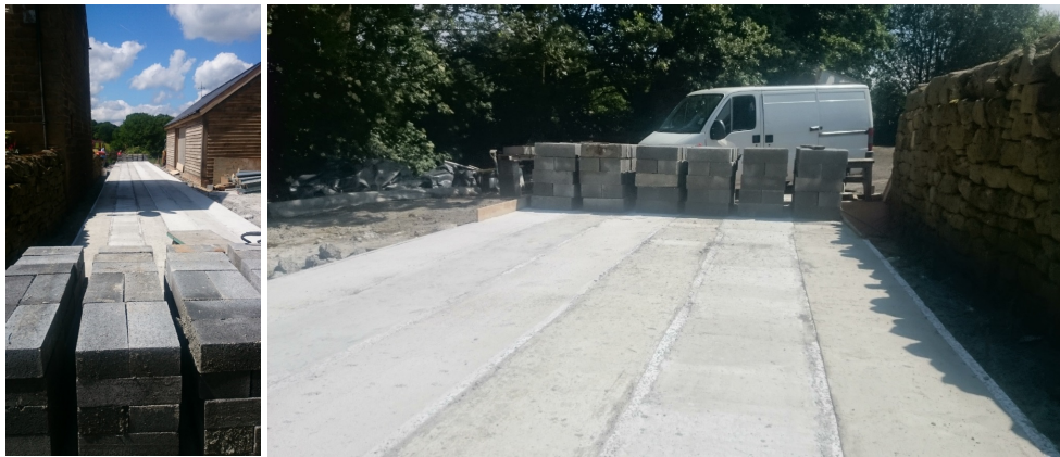
Figure 16 Finished concrete strips
