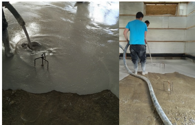
Figure 34 Casting of fibre reinforced screed
