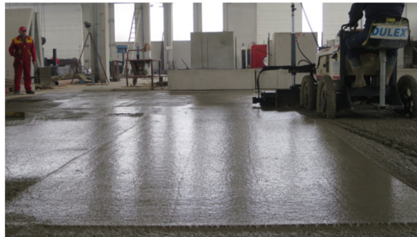
Figure 29 Laser-guided levelling
