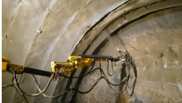
Figure 31 Spraying the 300mm-thick concrete layer
