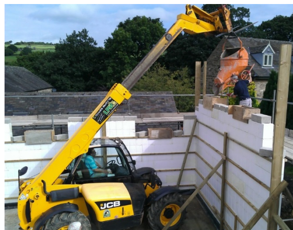
Figure 36 Casting concrete into screen-grid ICF moulds in constructing a high wall, with supporting scaffolding
