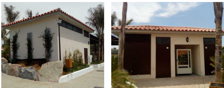
Figure 28 Finished sanitary hub
