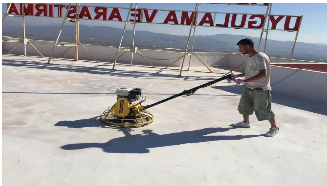
October 2016 – 3. phase insulation works / 5 mm paste blend application
