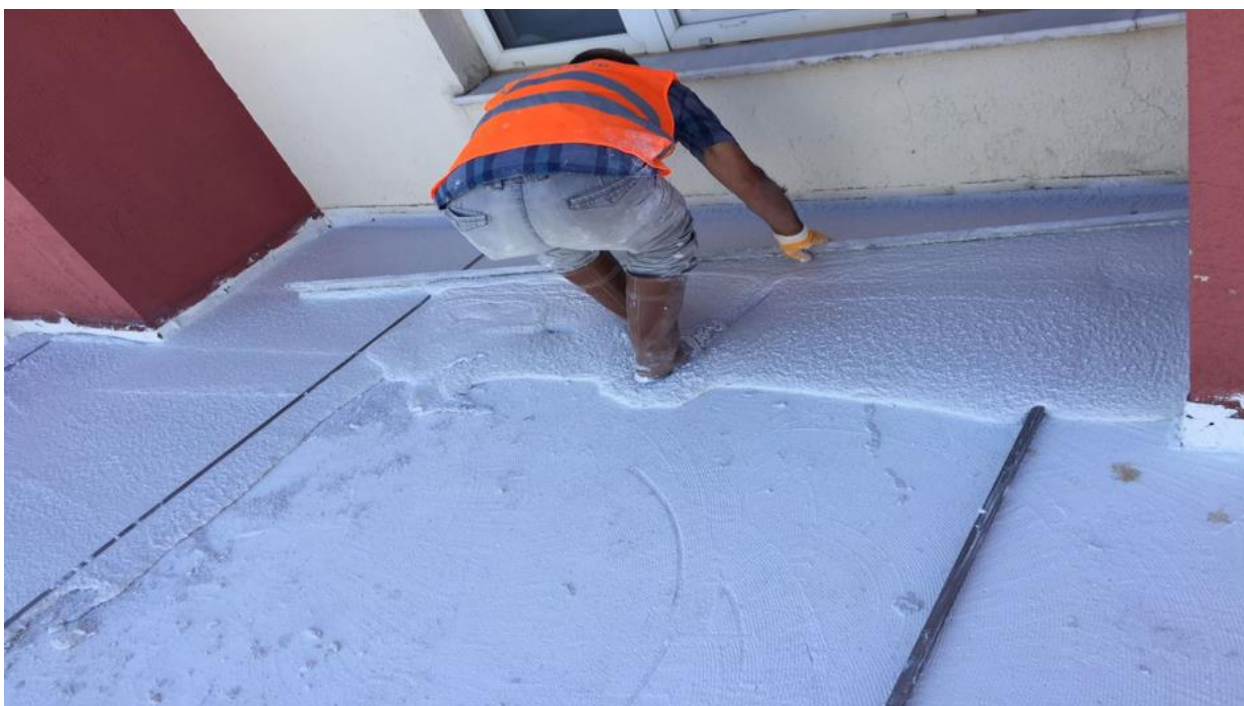
October 2016 - 2. phase insulation works / 26 mm main blending on the roof floor
