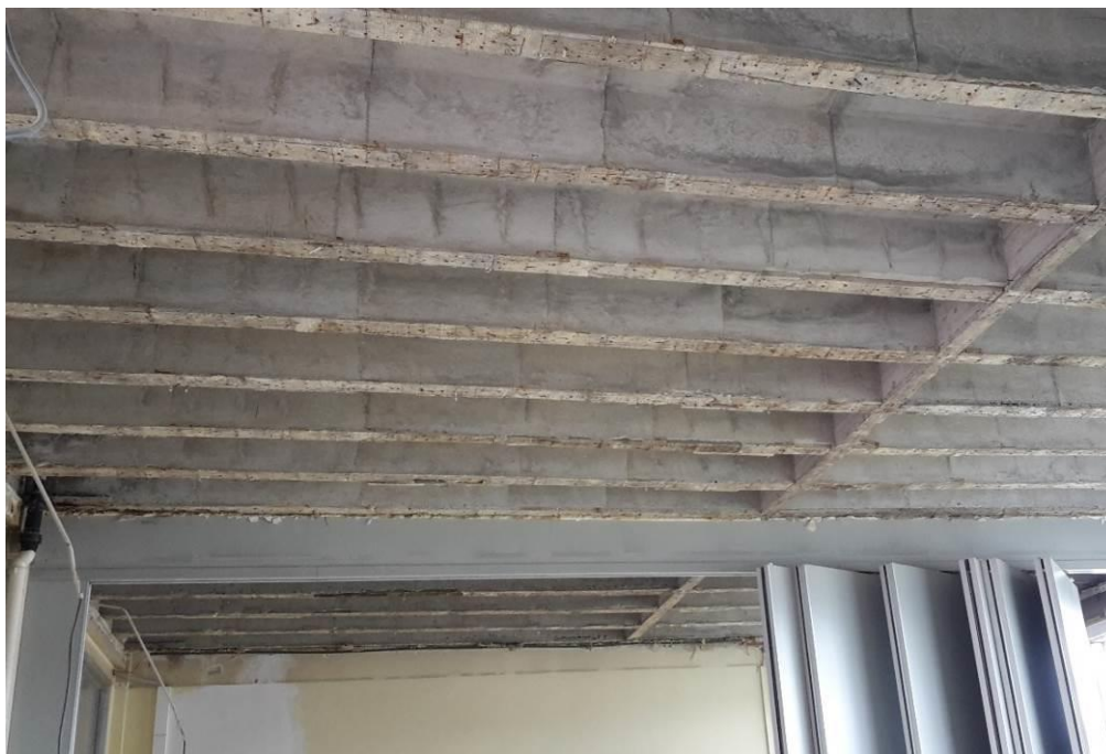
May 2016 - Dismantling of the ceilings for the PCM-based installation
