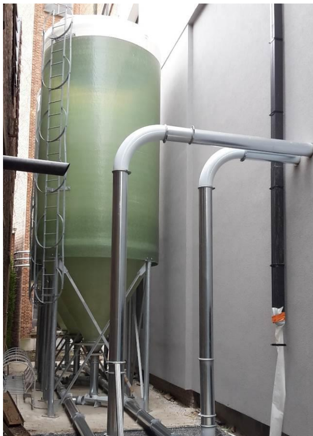
March 2017 – Storage of pellets in 3 silos
