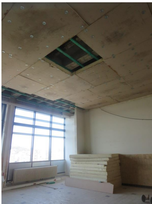
PIR foam panels with embedded PCM installation works in Liège.
