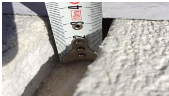
October 2016 – height control of the insulation layers
