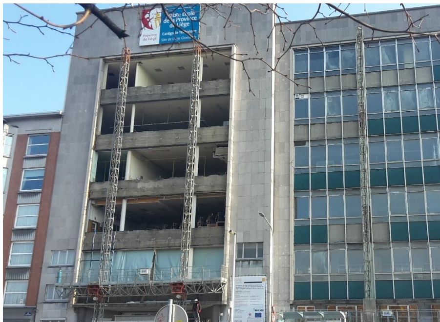
February 2016 – Dismantling Curtain Wall A
