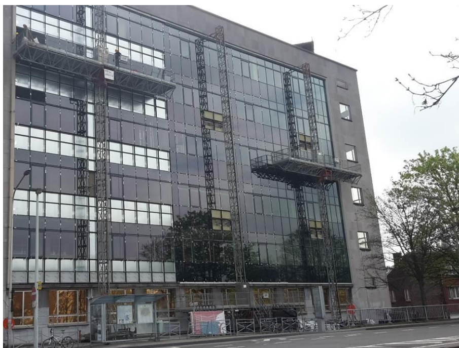
April 2016 – Rebuilding Curtain Wall B
