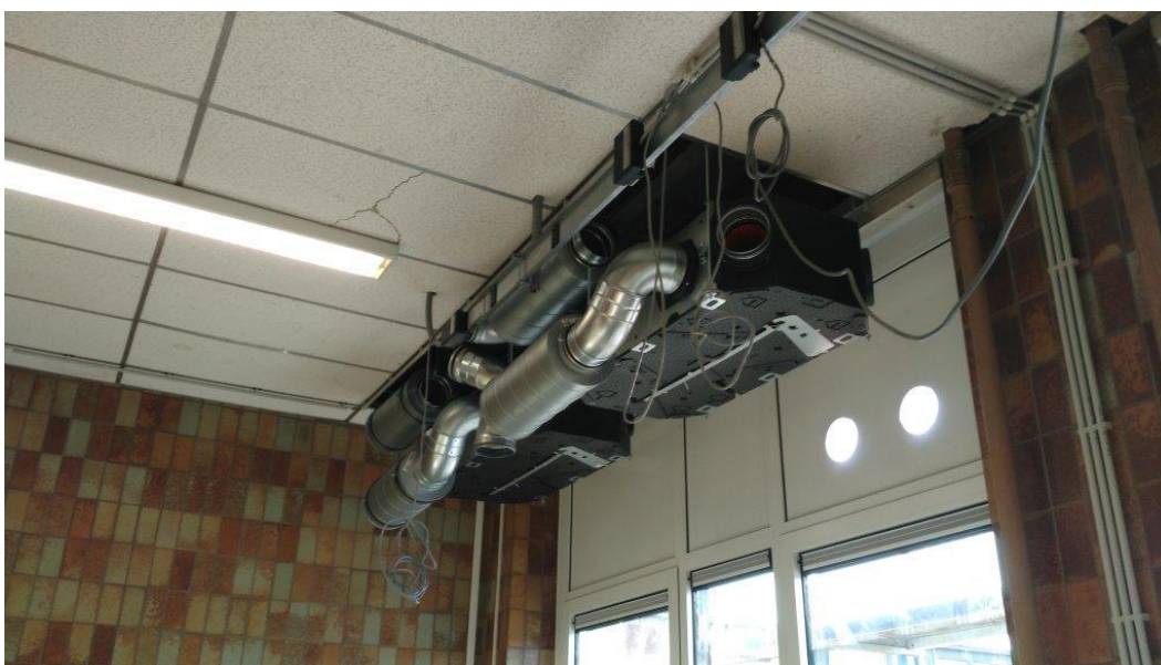
GRECOM first double flow unit installed at MONTH 36.
