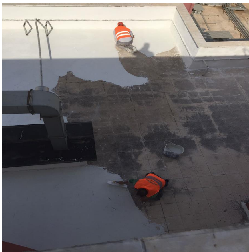
October 2016 – 1. phase insulation works / notching & 3 mm main blend application on the roof floor
