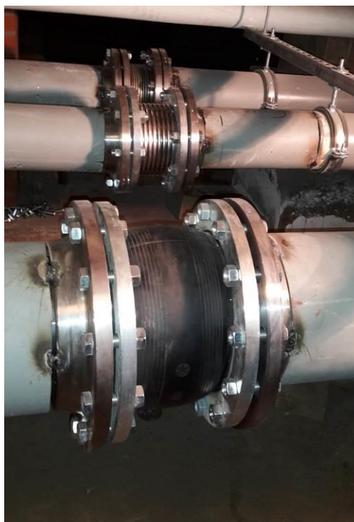
August 2017 – Expansion joints between old and new heating rooms
