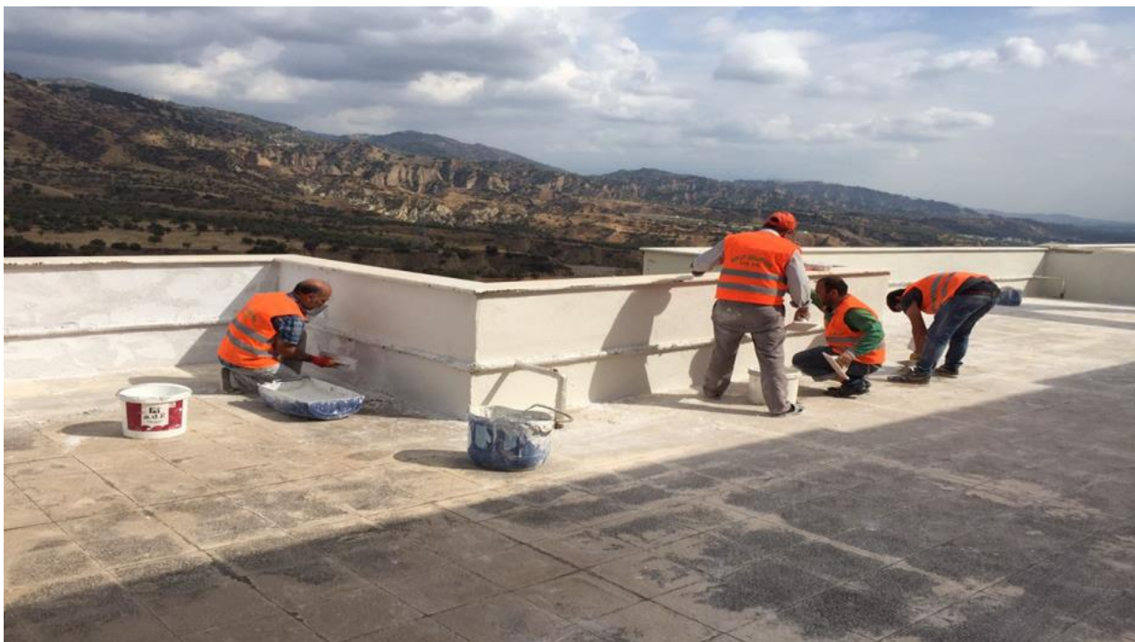
October 2016 - Insulation works on the upstand
