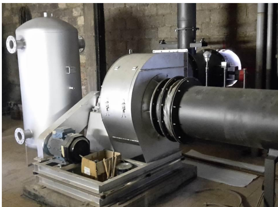
April 2017 – Chimney extractor and storage tank for thermal oil
