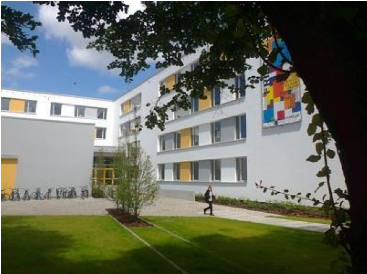
A transformed image of the Frieda 23 building
